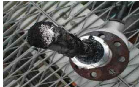
BWT removed from coker feed furnace for inspection
